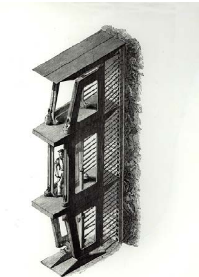
Figure 1-1 Brunel's iron frames used inside the tunnelling shield [51].
